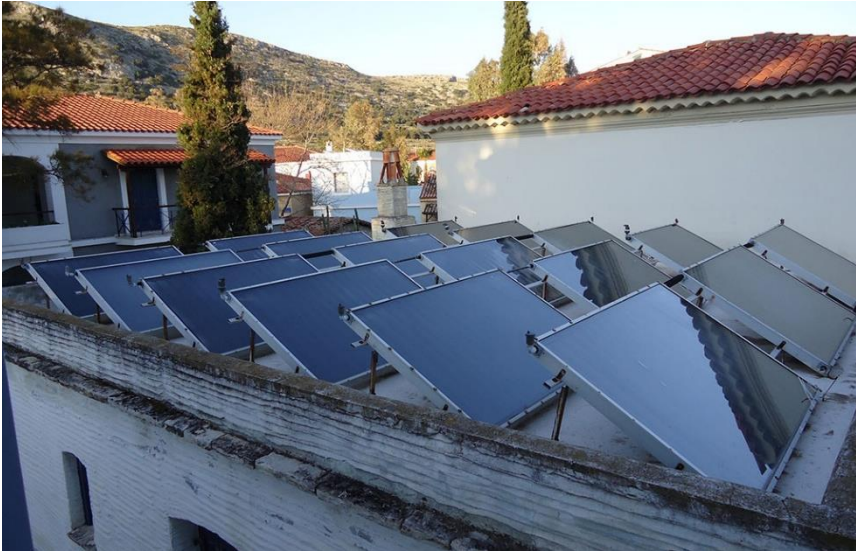
Figure 21: Solar panels placed on the rooftop of the hotel building
