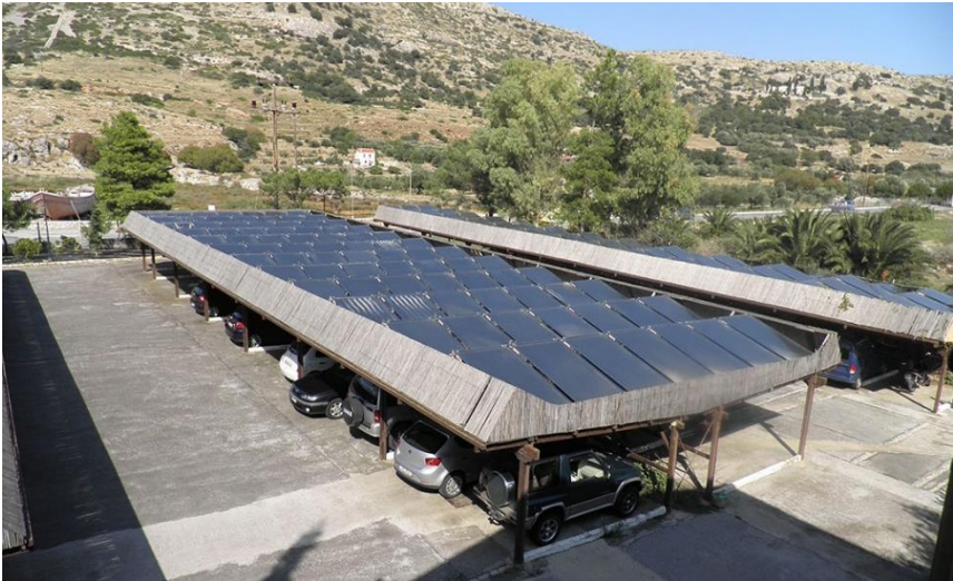
Figure 20: Solar panels placed on top of the parking lot
