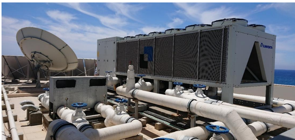
Figure 15: Six-pipe simultaneous chiller installed on the rooftop of the hotel
