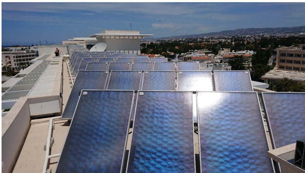
Figure 16: 45 solar thermal panels installed on the rooftop of the hotel
