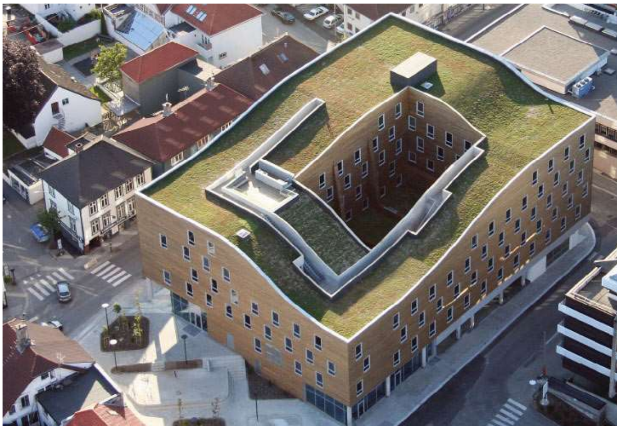
Figure 23: Photo of a green roofed resort
