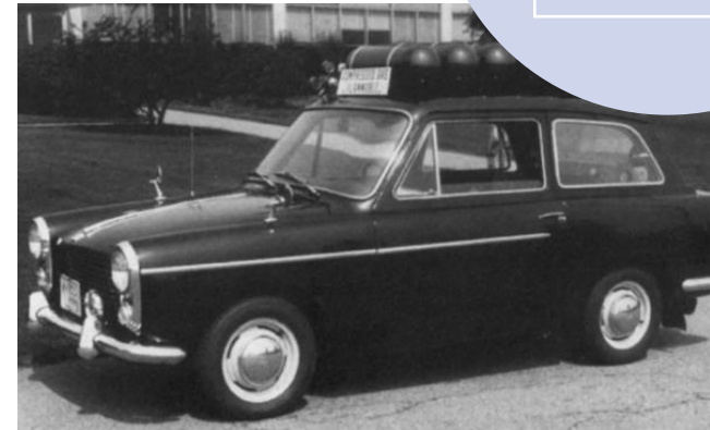
Austin A40 with a hydrogen fuel cell. He used the vehicle as his personal transportation for over three years (1970)
