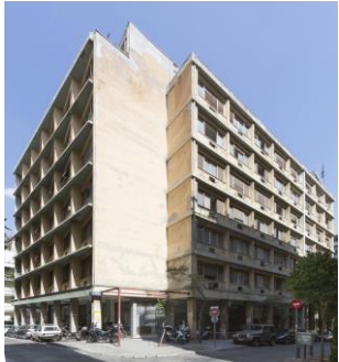
From ...no insulation
