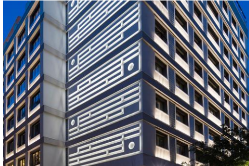
To ...high external thermal insulation and thermal windows
