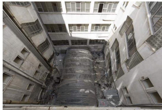
From ...uninsulated external atrium
