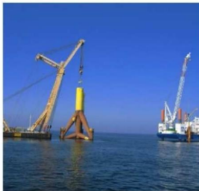
Heavy-lift crane ship on site
