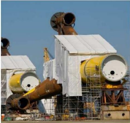
Tripods being welded
