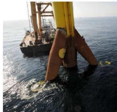
Tripod foundation lowered to seabed
