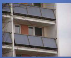
Solar collectors act as balcony railings of the building, China
