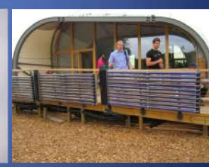
Solar collectors act as balcony railings of the building, China
