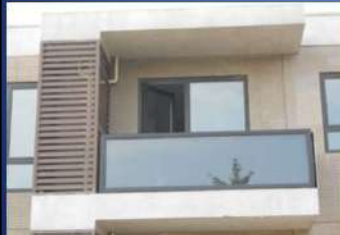
Solar collectors act as balcony railings of the building, China
