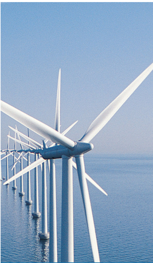
Offshore wind energy
